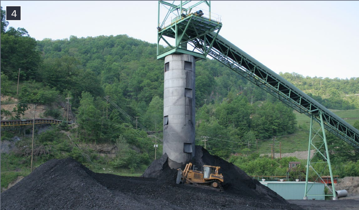
4. Bulldozer working ICG's coal stacker preparation plant near Raven, KY.
