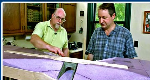
Installing roadbed and fascia
