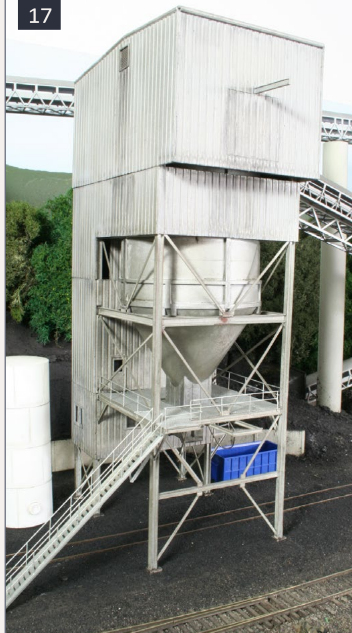
17. The finished fast loader from the left front.
